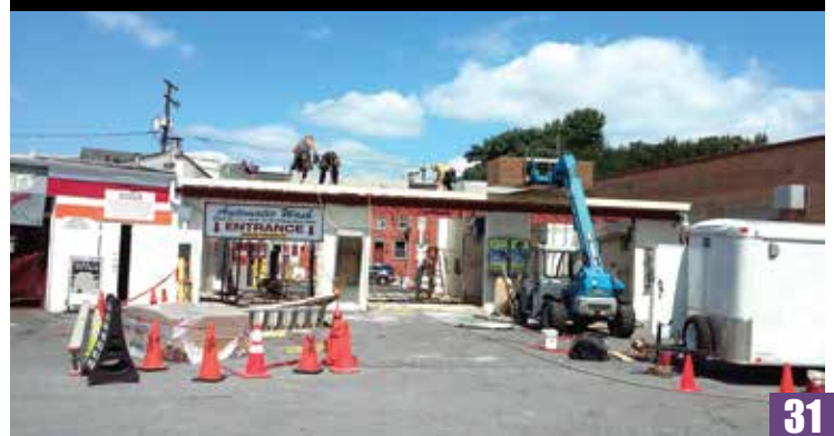
The roof and beams over the wash were replaced in the summer of 2016.
